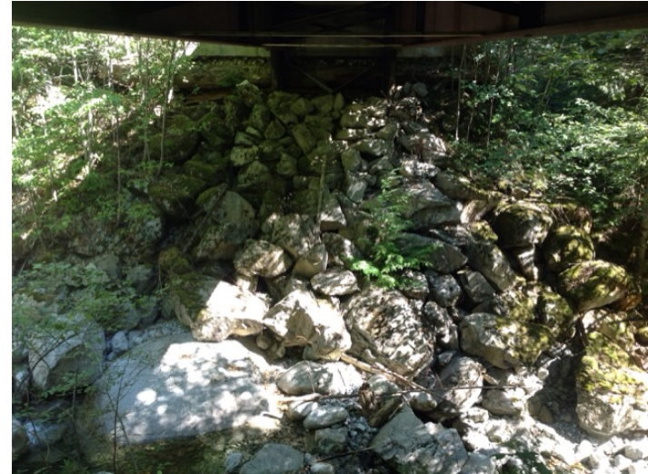
Left Bank Abutment when facing downstream
